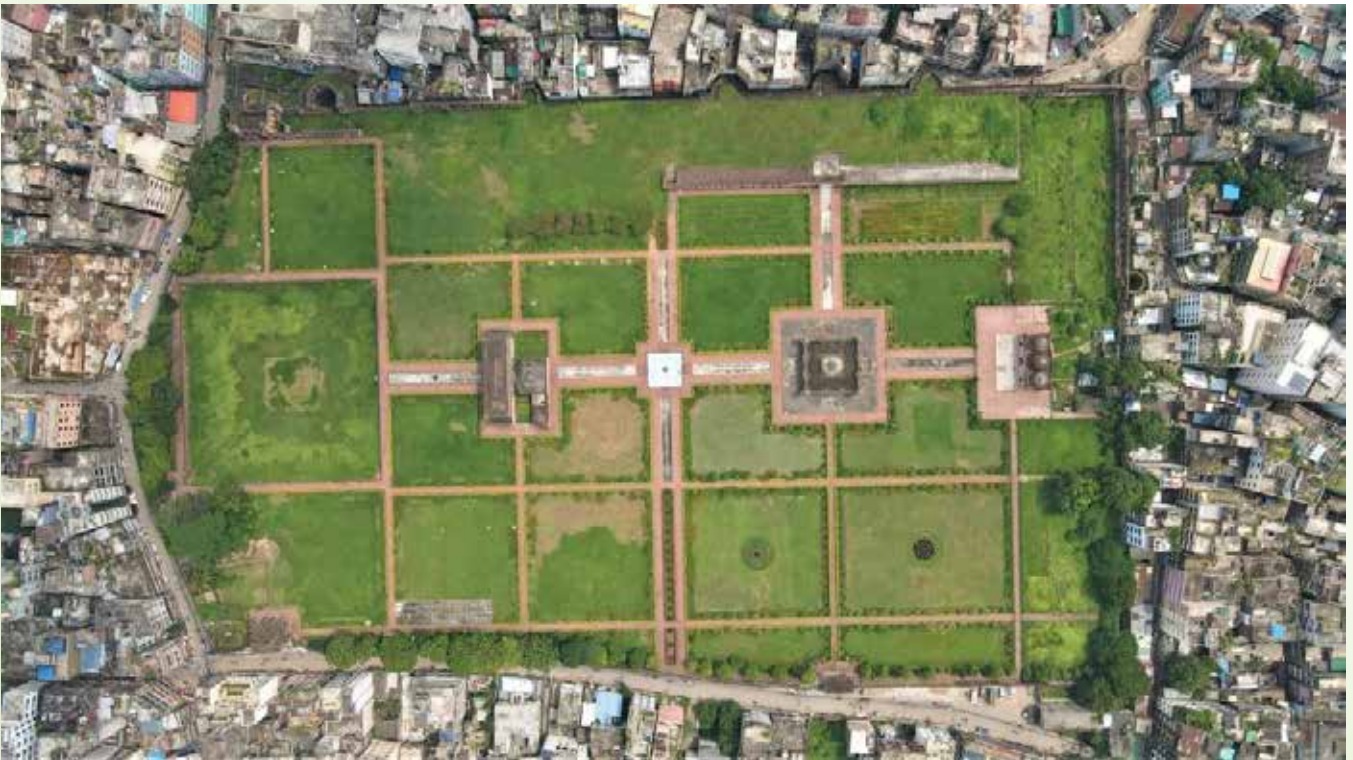
Aerial view (altitude 329.4 m) of Lalbagh Fort
